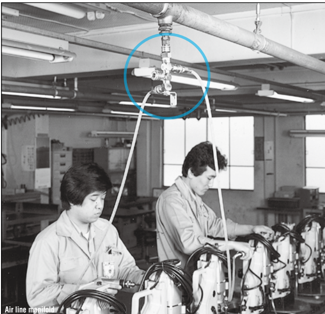
Air line manifold
